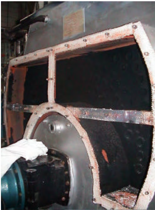
Tube Condition Before Installation
