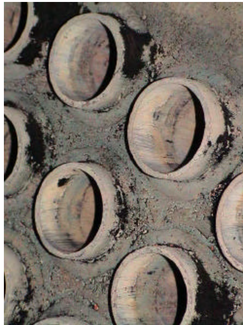
Tube Condition After Installation
